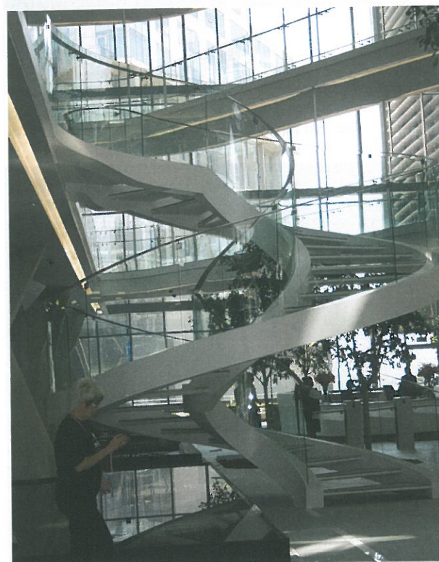
115 West Street's sharply curved spiral glass-walled steel staircase features an exceptionally tight internal glass radius
