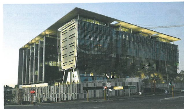
Twenty 9 metre high, sloping, tapering concrete columns – weighing 16 tons each – had to be secured in place for two weeks before the concrete slab on top could be cast and the formwork released. Six of the columns have a side protruding bridge support column
