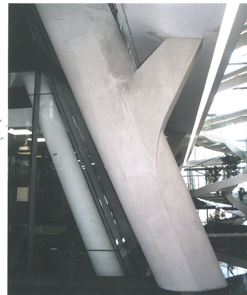
Twenty 9-m-high, sloping, tapering concrete columns weighing 16 tons each had to be secured in place for two weeks before the concrete slab on top could be cast and the formwork released. Six of the columns have a side-protruding bridge support column.
